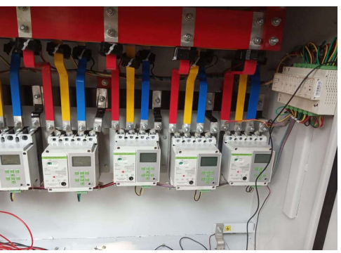
Smart MCCB Mobile Operated Panel
