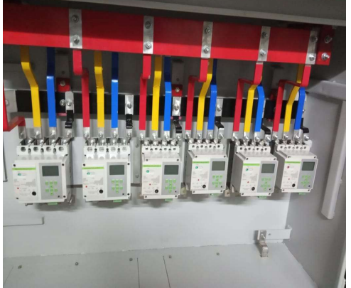
Mobile Oprated Smart MCCB Control Panel
